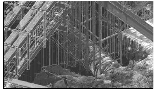
(a) Point cloud by 3D laser scanner
